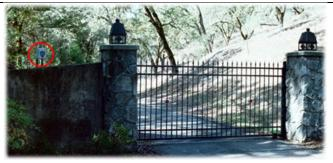
A properly installed C2E box is clearly visible to approaching traffic.
