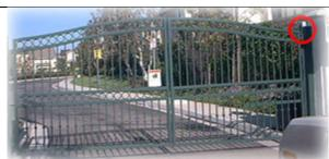
This is an improper installation. The box does not face oncoming traffic. The indicator light cannot be seen by emergency personnel.
